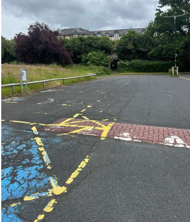
Photograph 4: School Drive Car park
