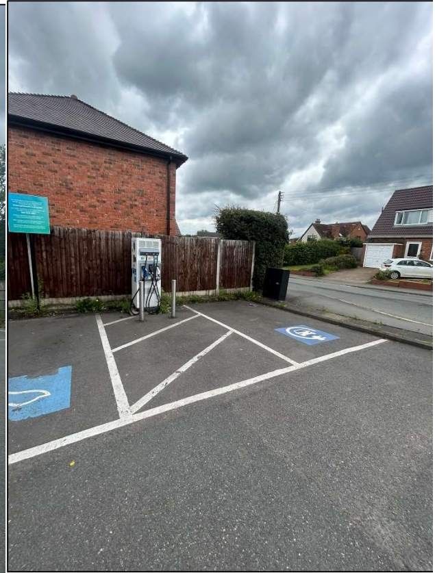
Photograph 11: Catshill Car park
